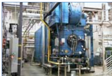
Energy Recovery Boiler
