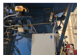
Central Plant: Actuator & linkage air damper for boiler
